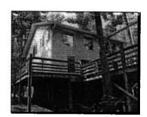
here is a beautiful post and beam constructed house in the woods of western Orange County that is insulated with bales of straw. No, the straw is not stacked around the outside of the house, but baled and placed on a moisture barrier at least six inches above the final exterior grade and hold securely in place by two #4 rehar pinning each bale to the foundation. Subsequent bales also have two rebar holding them securely in place.
